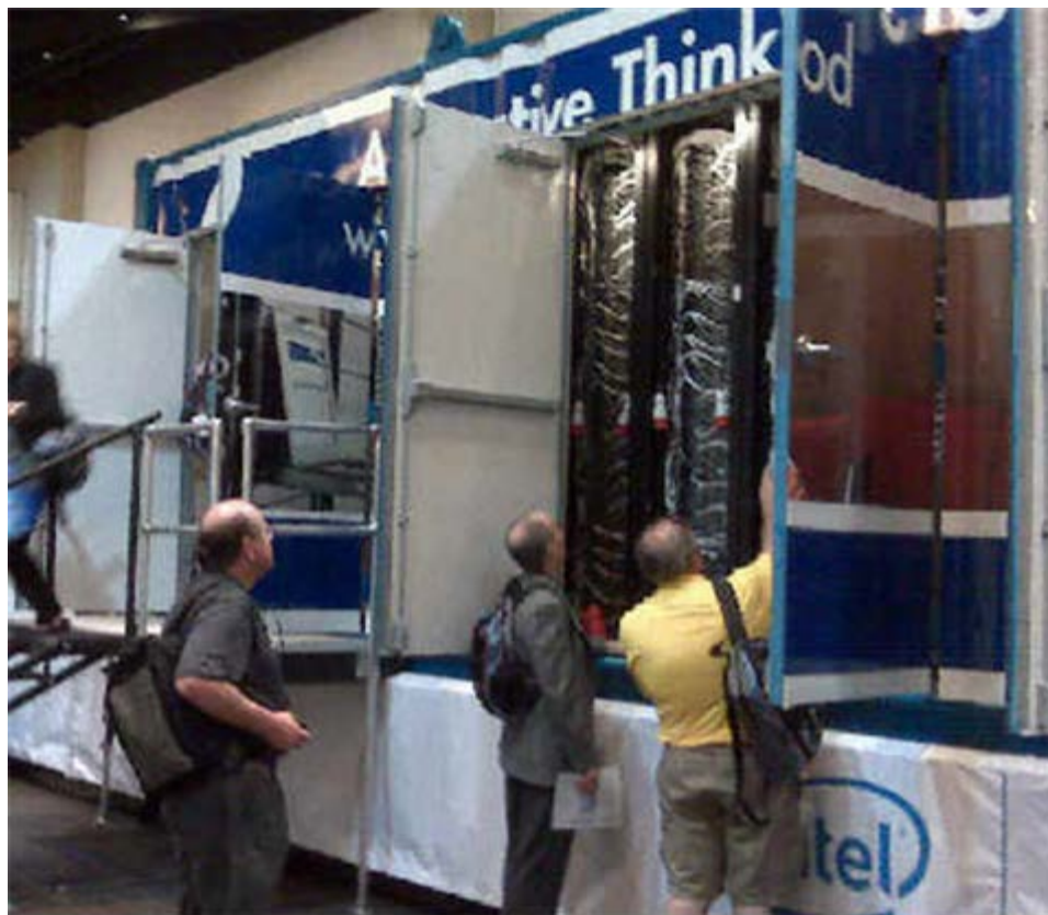
IT folks checking out the wiring behind the racks.
